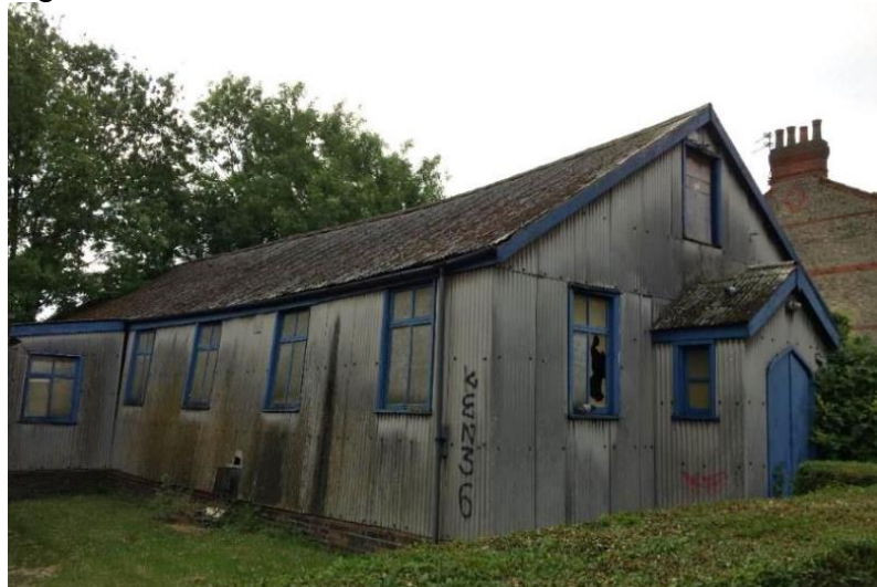
Figure 4 – Iron church hall
